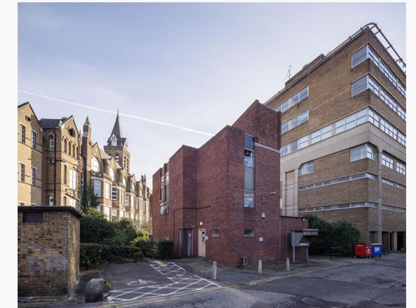
The Ely Building (centre) viewed from within the site with the Holborn Union on the left and Furnival on the right
