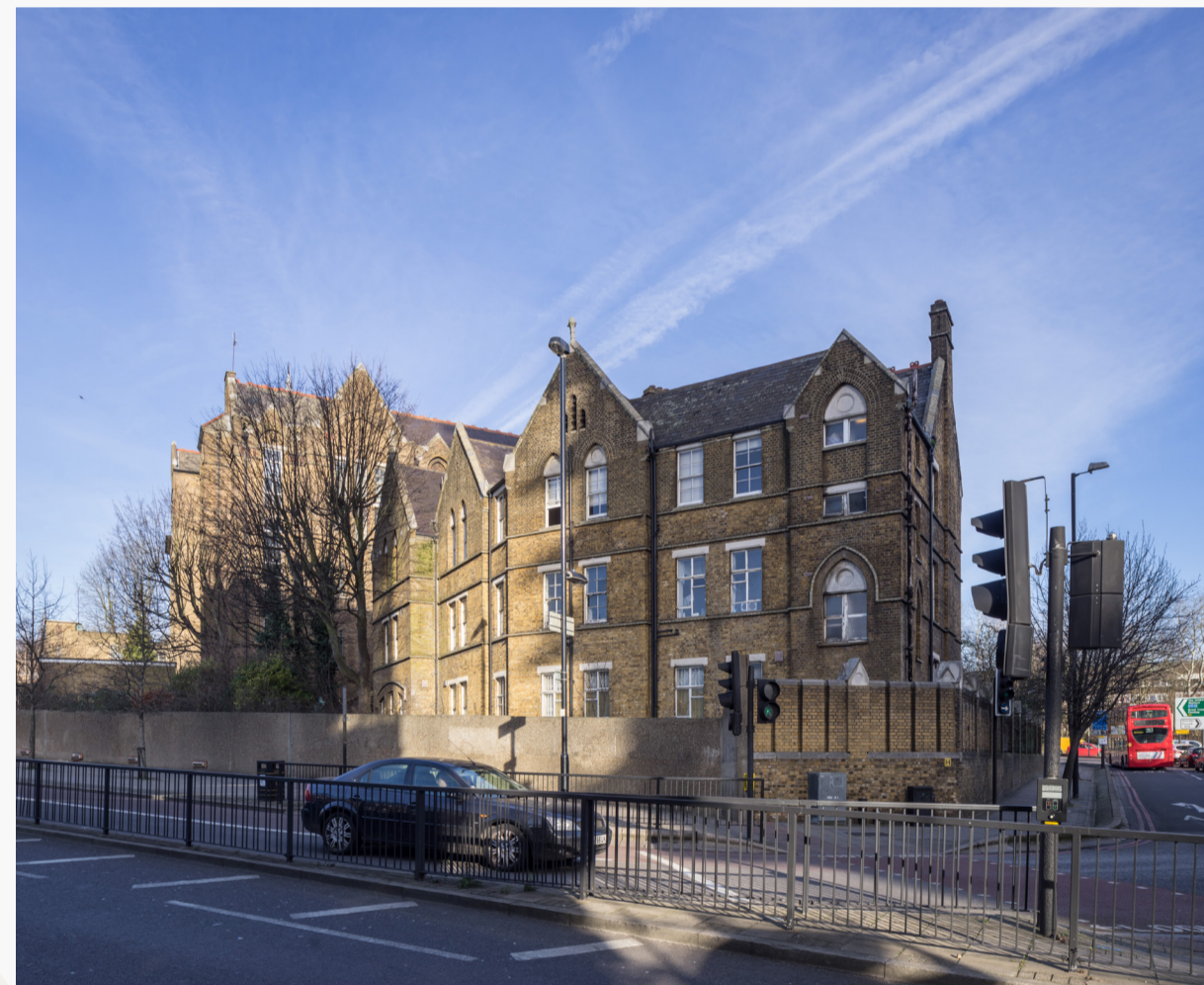
The Clerkenwell Building on the southern tip of the site viewed from Highgate Hill
