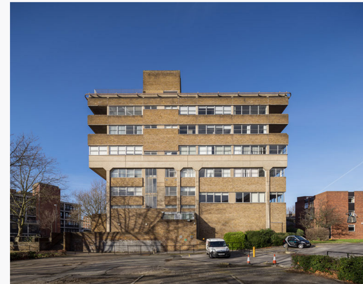
The Furnival Building viewed from within the site
