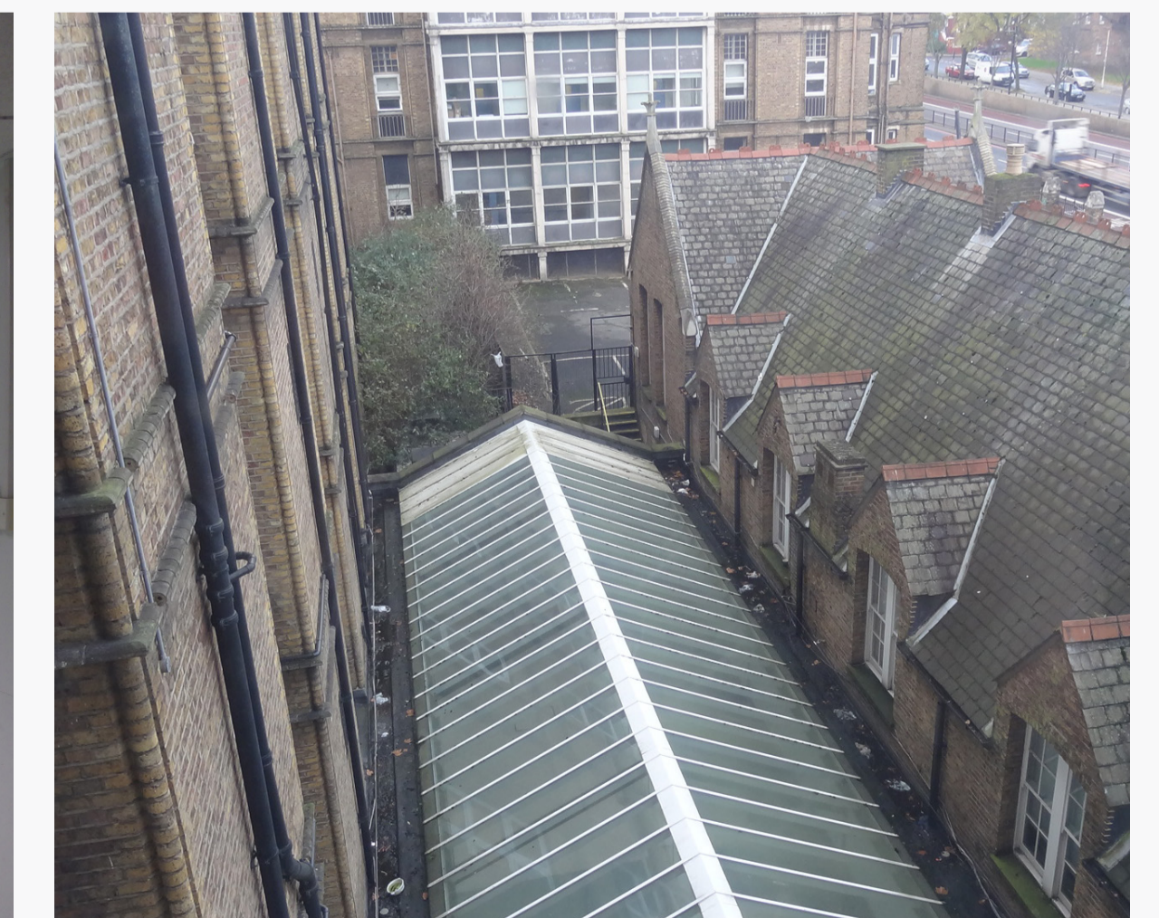
Glazed courtyard at the centre of the Holborn Union Building
